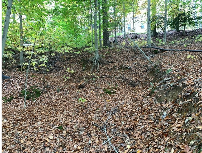
Site 7, Photo 5: Severe Slope Erosion (Southwest toward 113 Little John Road)
