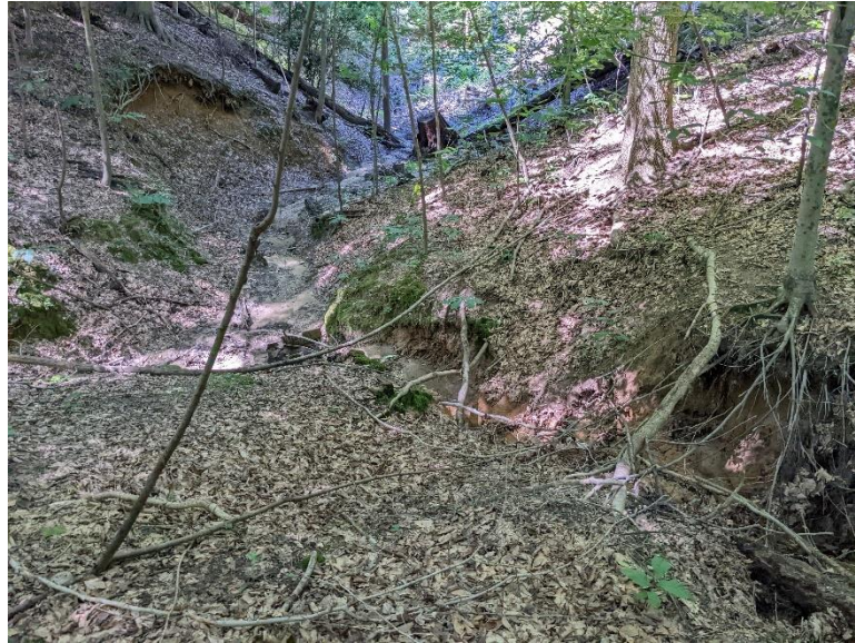
Site 5, Photo 5: Bank Erosion (Looking Downstream (West))
