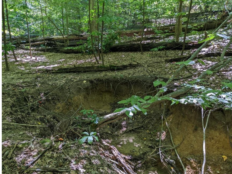
Site 7, Photo 1: Channel Erosion (Looking Upstream (Southeast))
