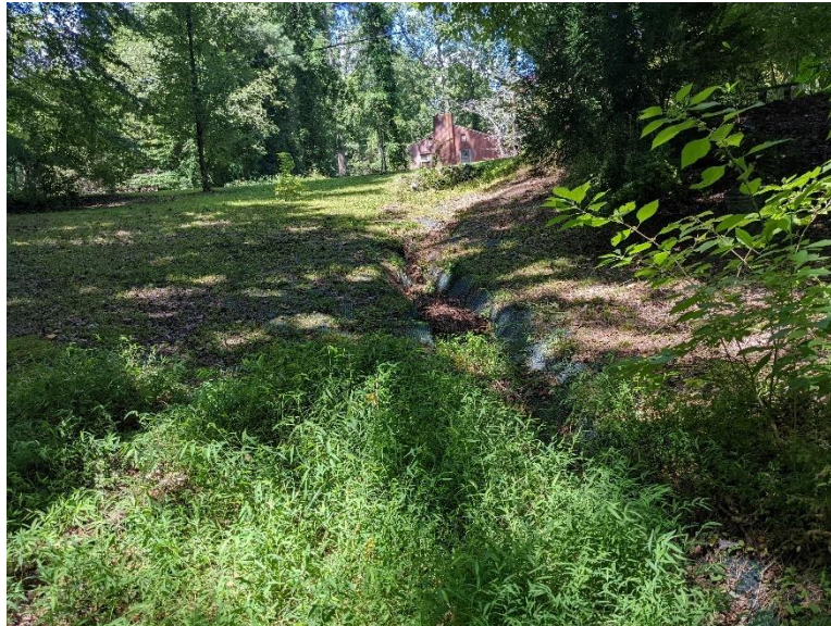
Site 4, Photo 1: Existing Geotextile Lined Channel from East Queens Drive (Looking Upstream (West))
