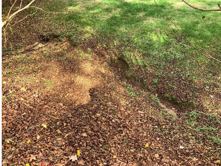
Site 2, Photo 1: Erosion on the Northeast side of Horseshoe Drive
