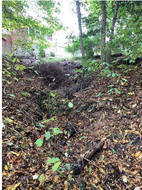
Site 4, Photo 5: Slope Erosion behind 266 East Queens Drive (Top of Slope, Looking North)
