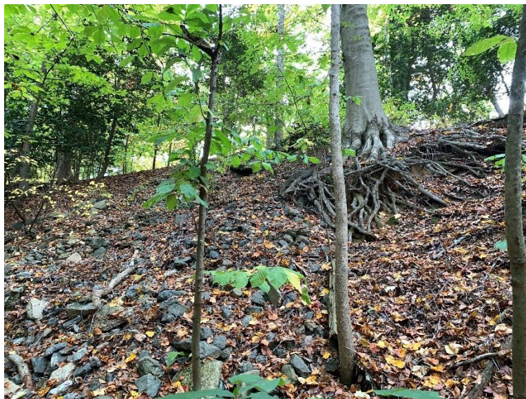
Site 6, Photo 4: Existing Rip Rap Slope Stabilization (Bottom of Slope, Looking Southwest)
