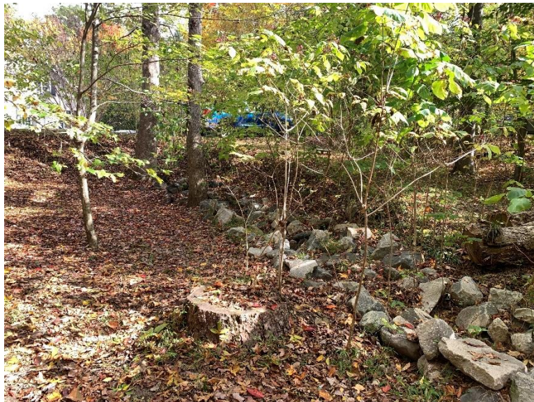
Site 2, Photo 2: Existing Rip Rap Channel (Looking Upstream (Northeast))
