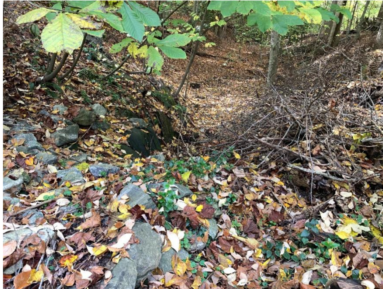
Site 2, Photo 3: End of Existing Rip Rap Channel (Looking Downstream (Southwest))
