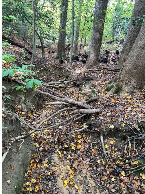
Site 1, Photo 5: Continuation of eroded ditch (Looking Downstream (West))
