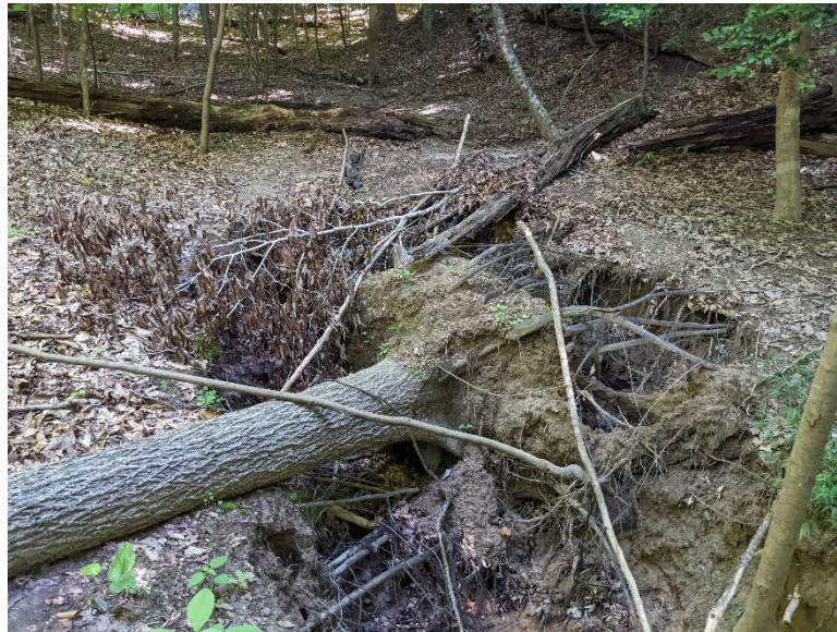
Site 5, Photo 3: Severe Erosion / Fallen Tree (Looking Upstream (East)) (Aug. 2022)
