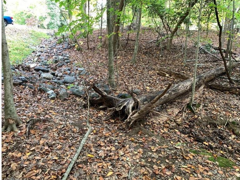
Site 5, Photo 1: Existing Rip Rap (Looking Upstream (East toward Nottingham Road))
