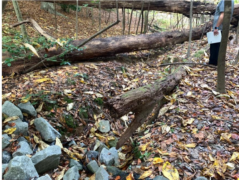
Site 8, Photo 3: End of Rip Rap (Looking Downstream into Woods)
