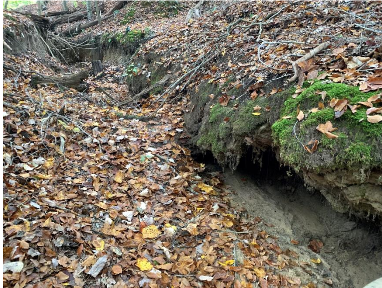
Site 4, Photo 9: Stream Erosion (zoom-in) (Looking Upstream (West))
