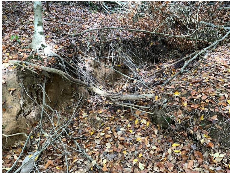
Site 5, Photo 4: Severe Erosion / Additional Fallen Tree (Looking Upstream (East)) (Nov. 2022)
