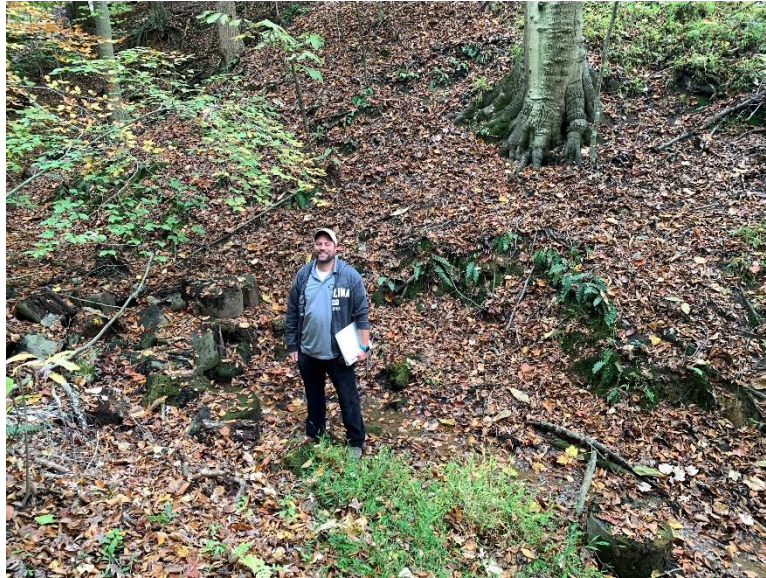
Site 3, Photo 3: Slope Erosion behind 110 Willoughby Drive (Looking Northeast)
