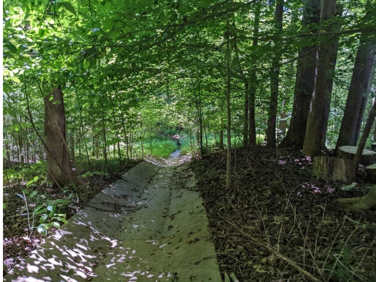
Site 10, Photo 1: Concrete Swale from Cambridge Lane (Looking Downstream (Southwest))
