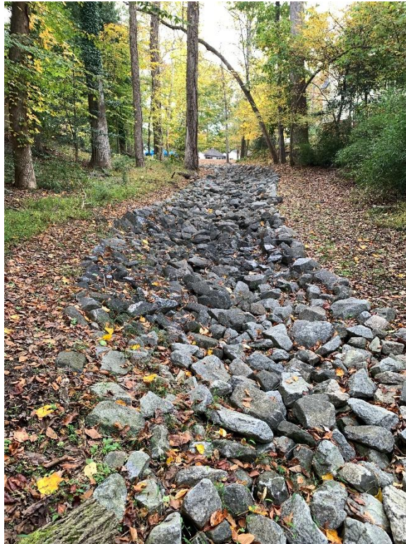
Site 8, Photo 1: Existing Rip Rap (Looking Upstream to Copse Way)
