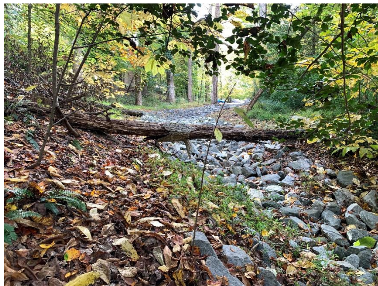
Site 8, Photo 2: Existing Rip Rap (Looking Upstream to Copse Way)
